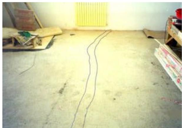
Figure 3: The position of tubes was marked in chalk on the floor surface.
