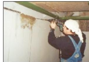
**Sealing the crack with wet seal grout**
