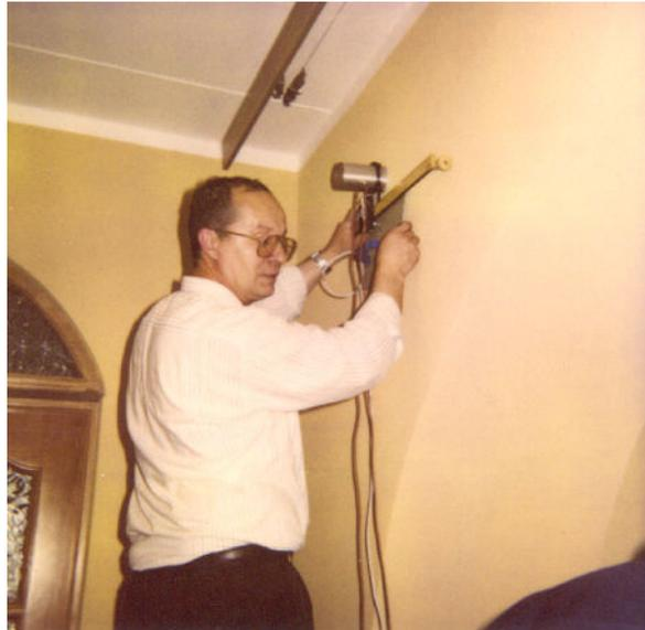
Fig. 3. An operator with the RASCAN radar during the sounding of the investigated arch
